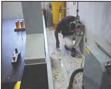
11. Application of Joint Filler V-100 Epoxy
