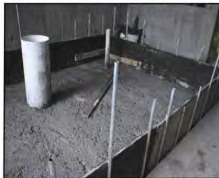
8. Inertia block concrete placed
