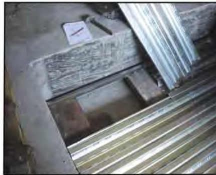
5. Setting of underlayment decking to support foundation
