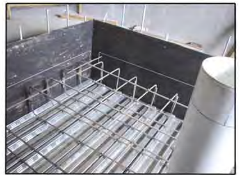
6. Reinforcing rebar cage
