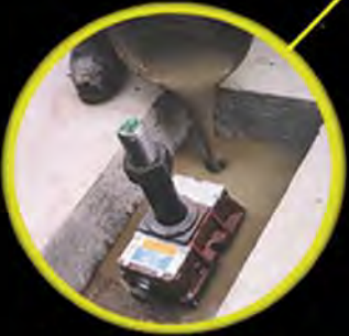
Advanced Grouting Techniques
