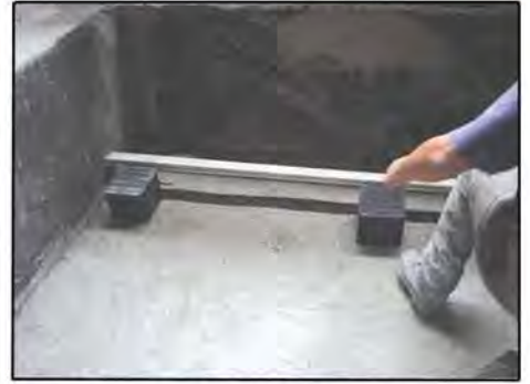
3. Placement of UNISORB GK Foundation Isolation Blocks
