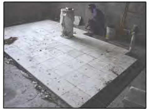
9. Granite tile installed
